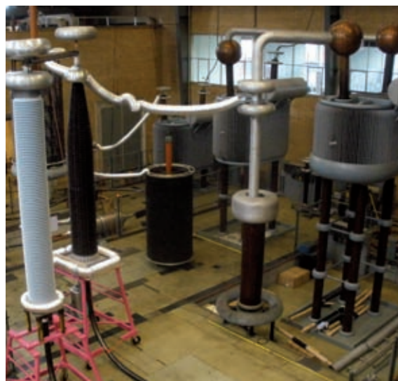
HV cascade transformers up to 900 kV, HRL Delft.
