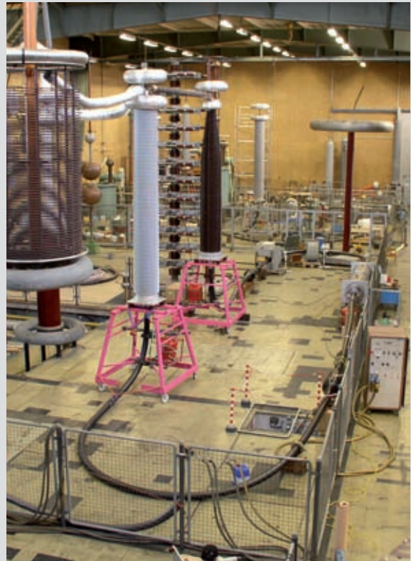
Type Test on a 2500 mm 2 400 kV cable system, HRL Delft.
