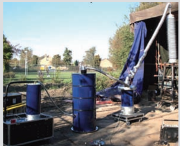
Set-up of the DAC 150kV system during a test on-site
