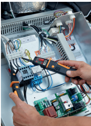
Measuring voltage on a compressor.
