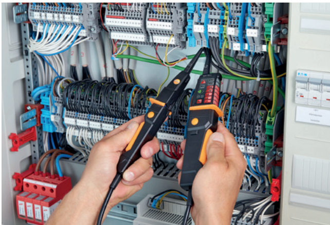
Measuring voltage in a switching cabinet.
