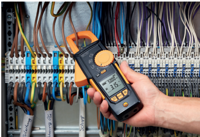
Measuring current in a switching cabinet.
