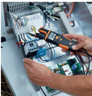
Measuring voltage on a compressor.
