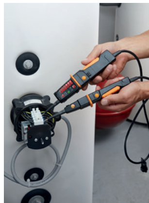
Measuring voltage on a boiler.
